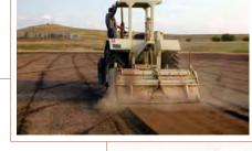
Following the installation of the amendments, the field was laser leveled in preparation for installation of specially grown athletic type sod.
