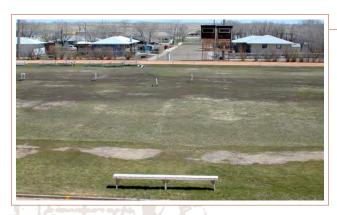
Steiner Thuesen PLLC was retained in the spring of 2002 to provide a renovation design for the field. Soils tests revealed a shallow root zone comprised of sand high in sodium with very little organic material. Additional tests revealed irrigation water with an extremely high salt content.
