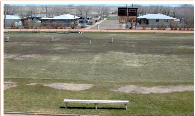
Steiner Thuesen PLLC was retained in the spring of 2002 to provide a renovation design for the field. Soils tests revealed a shallow root zone comprised of sand high in sodium with very little organic material. Additional tests revealed irrigation water with an extremely high salt content.
