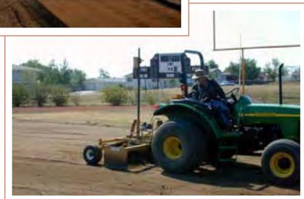
Following the installation of the amendments, the field was laser leveled in preparation for installation of specially grown athletic type sod.
